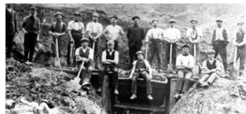
31. Littleworth Brickworks 1930s
