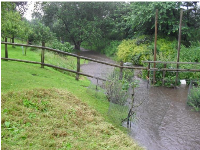
Figure 1: Flow down the railway cutting in Littleworth (during flood of July 2012).
