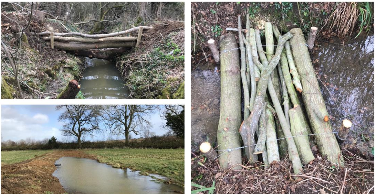
Figure 5: Example photographs of a leaky dam (top left), debris dam (right) and banded storage area (bottom left).
