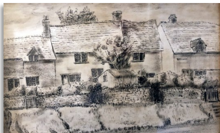
Cottages in Crown Square demolished in 1959/60. WW1 fatality Lawrence Thomas Johnson lived in 5, Crown Square
