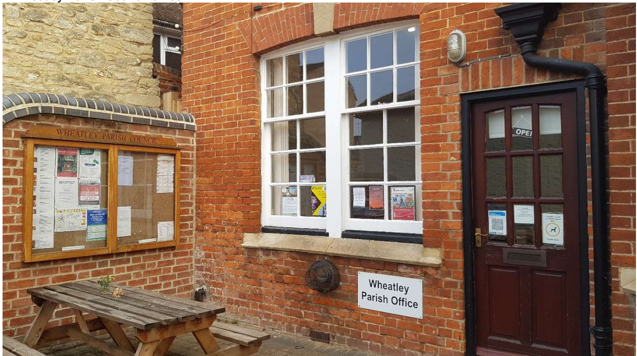
2 Wheatley Parish Council Office
