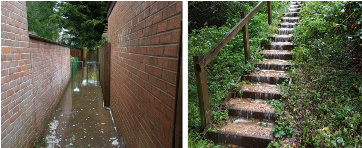
Figure 8 – Photographs of flooding in nature reserve and access footway (source; Wheatley Flood Group)
